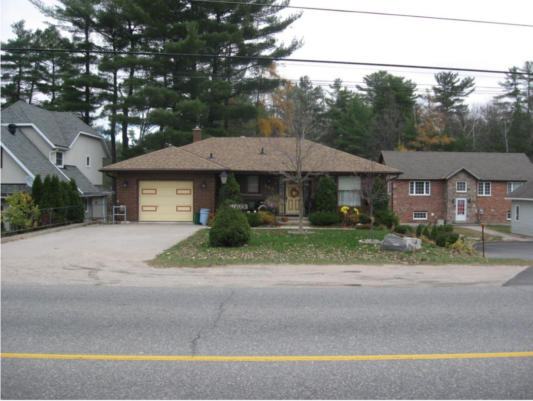
324 Bethune Drive N. Looking East
