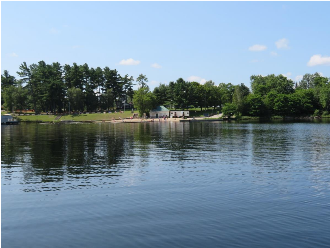
Gull Lake Park and Moonlight Bay Property Looking Southwest
