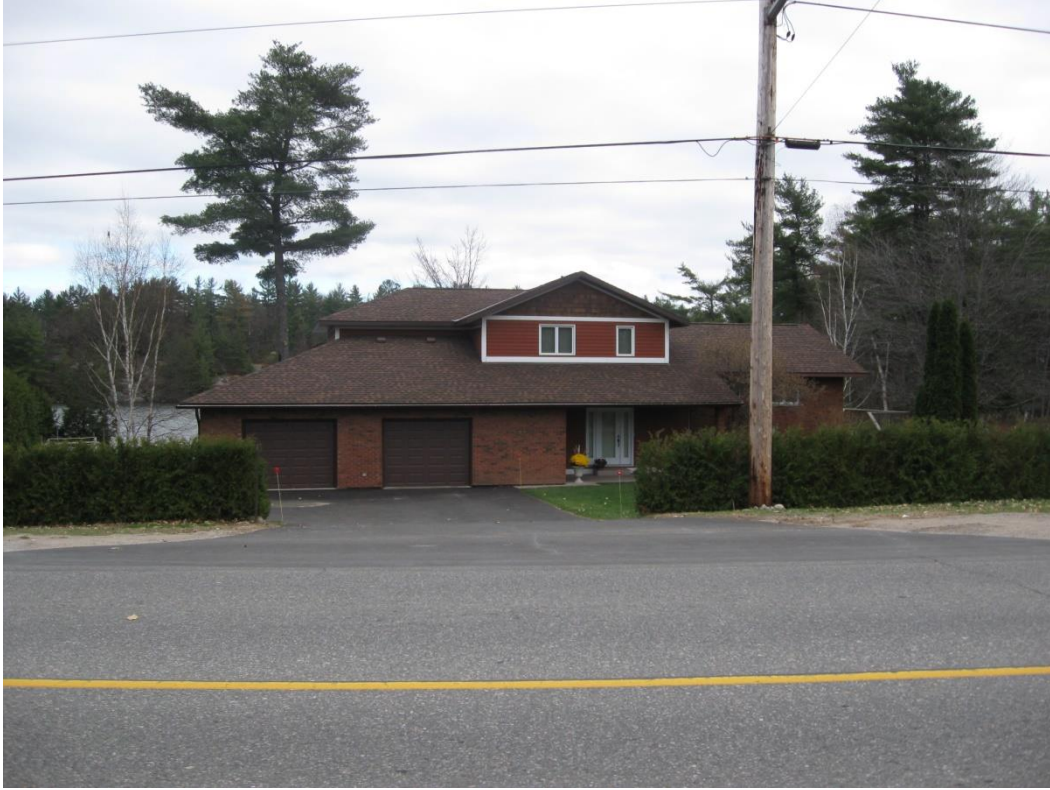
330 Bethune Drive N. Looking East
