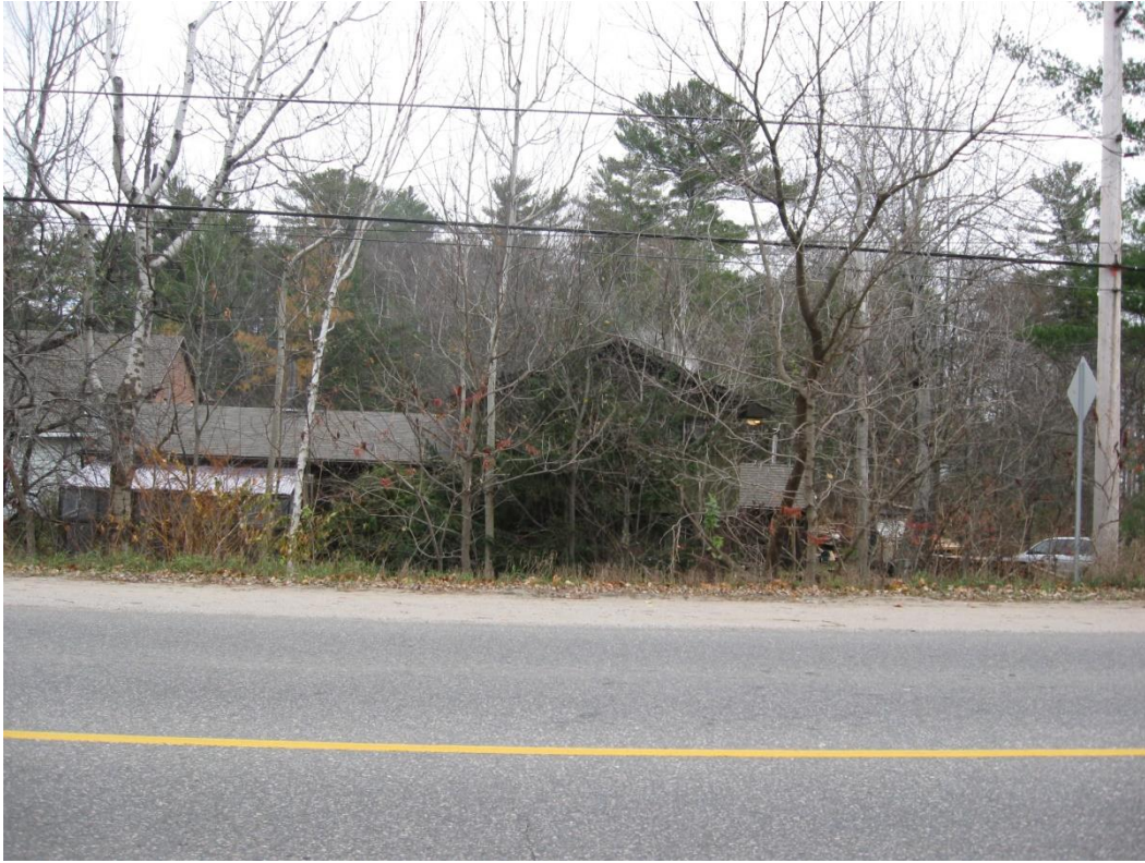
320 Bethune Drive N. Looking East
